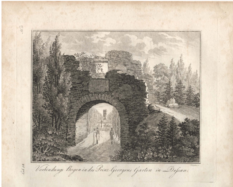
Fig. 28: Connecting bridge in the garden of Prince George, Dessau
