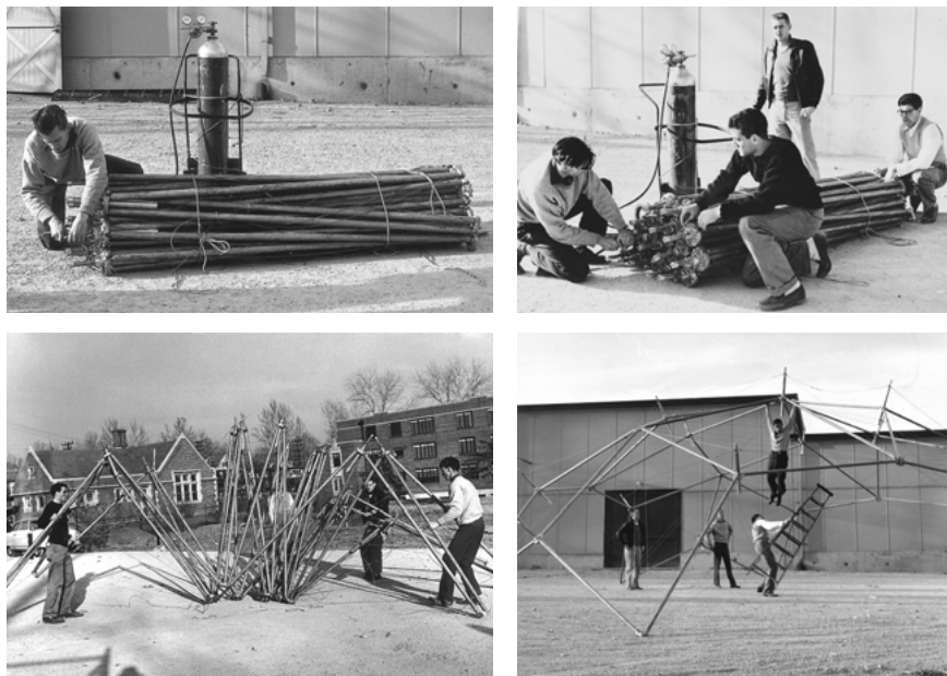
Fig. 2: Flying Seedpod. Washington University, St. Louis, 1953; A folding-out geodesic structure.
