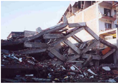
Fig. 1.5: Collapsed RC frame structure due to failure of beam-column joints, 1999, 7.2 Richter earthquake, Duzce, Turkey
