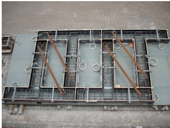
Fig. A.3: a) Specimen bracing, b) Formwork and bracing
