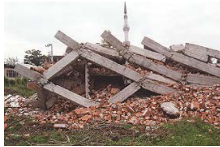
Fig. 1.6: RC frame structure was collapsed via failure of beam-column joints, 1999, 7.4 Richter earthquake, Kocaeli, Turkey
