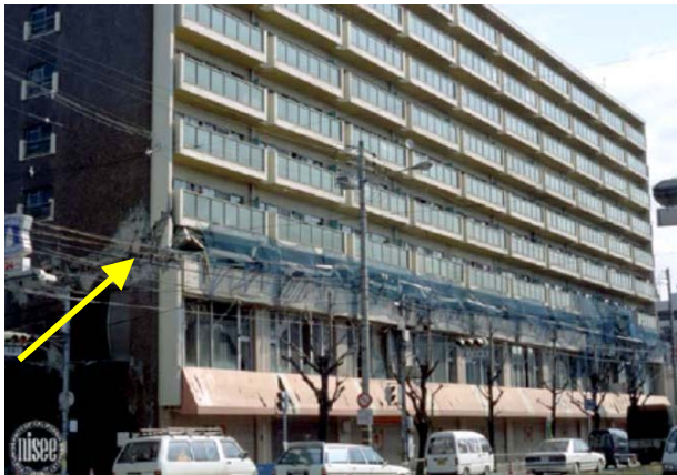
Fig. 3.2: Column sidesway mechanism led to 3 rd floor soft story collapse of reinforced concrete building in Nishinomiya, Kobe earthquake, Japan, 1995, Magnitude: 6.69 (Figure from USGS achieves)
