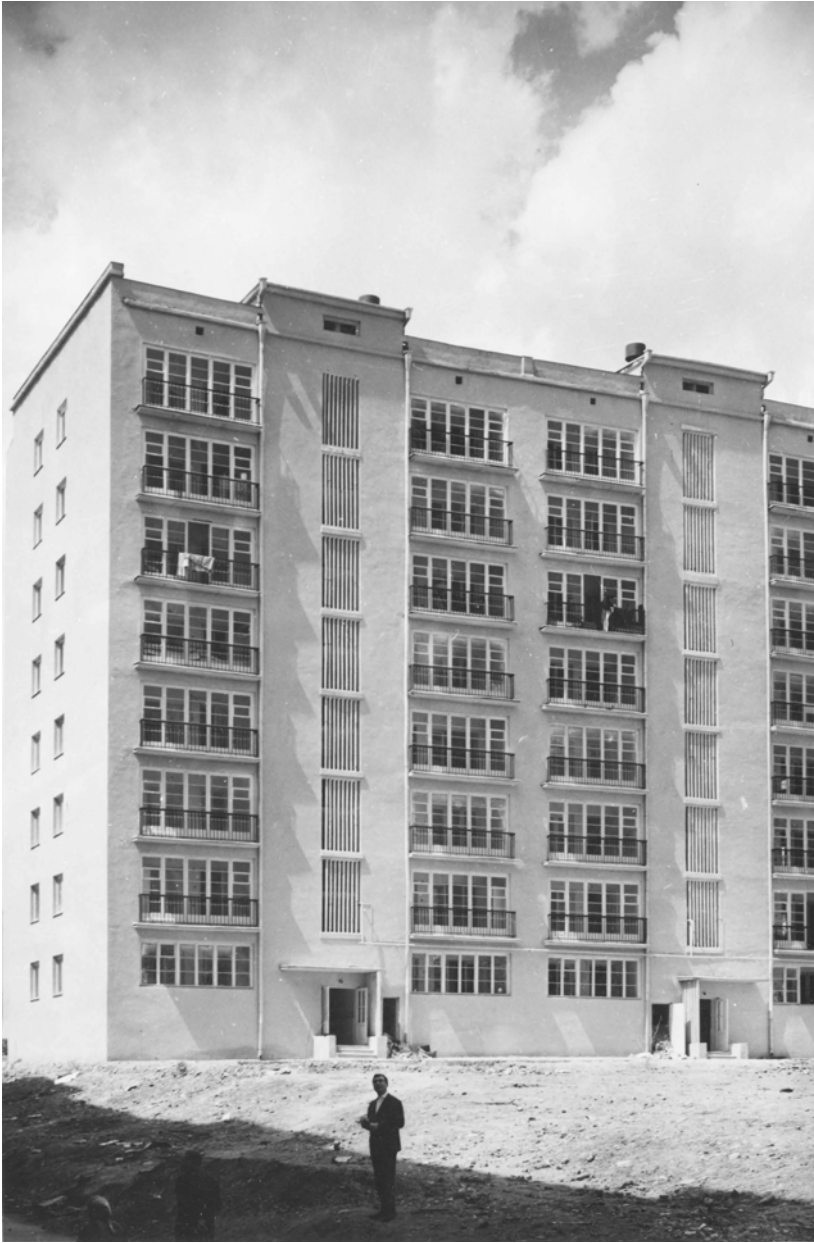
Figure 12: Eight-story residential building in Saburtalo, 1950s/1960s Source: Shota Kavlashvili's private archive, Tbilisi
