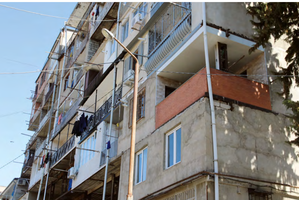
Figures 2, 3: Apartment building extensions (ABEs) in Vazha-Pshavela Block VI. The photo illustrates how each family has constructed its own extension. The resulting differences point to an unregulated construction process, highlighting the lack of standardized guidelines.
