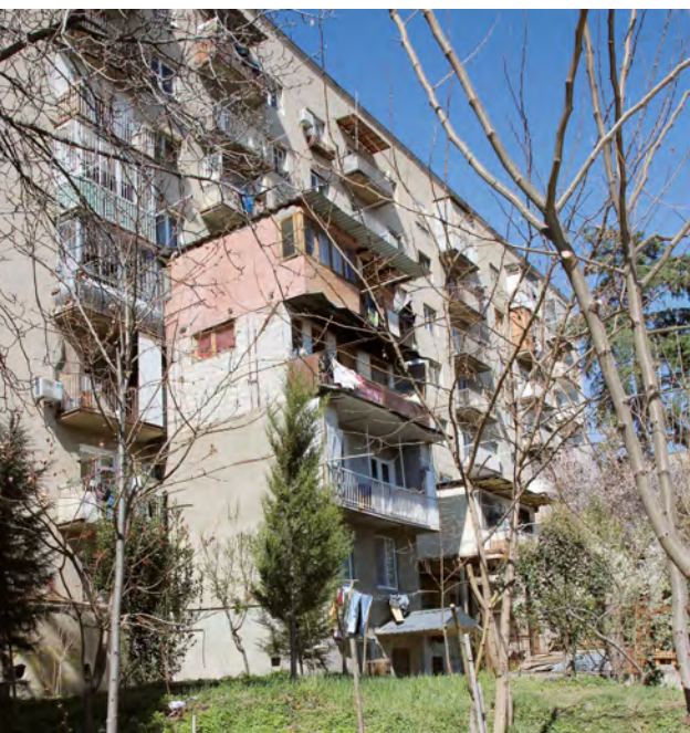
Figures 2, 3: Apartment building extensions (ABEs) in Vazha-Pshavela Block VI. The photo illustrates how each family has constructed its own extension. The resulting differences point to an unregulated construction process, highlighting the lack of standardized guidelines.
