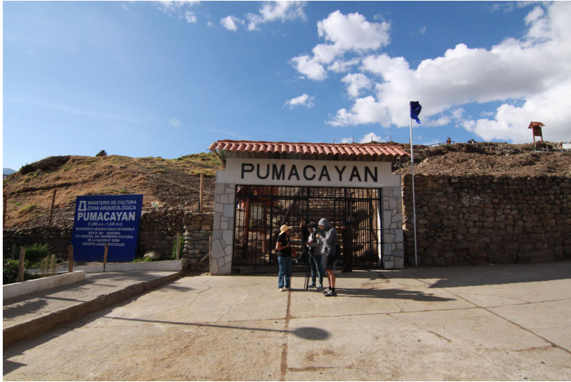
Figure 9: Pumacayán's main entrance of concrete and steel (Usón 2020)
