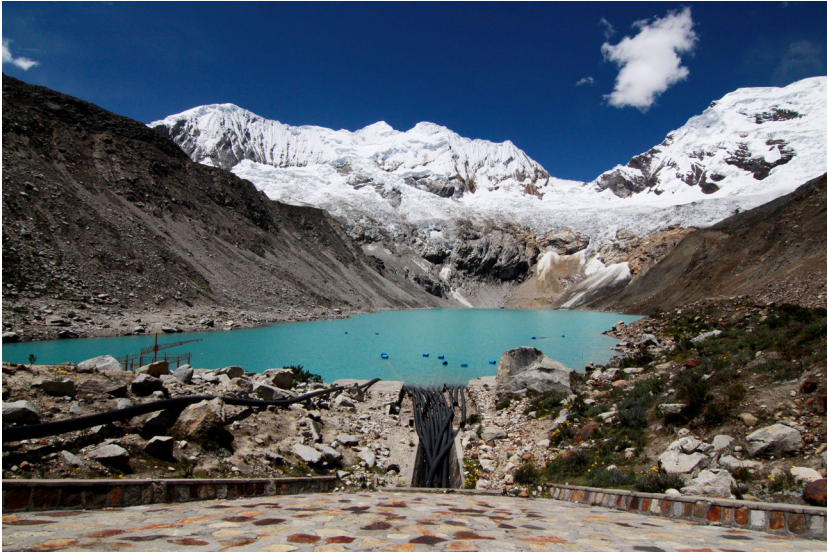
Figure 14: Syphons installed in Palcacocha, passing under the retaining wall (Usón 2020)
