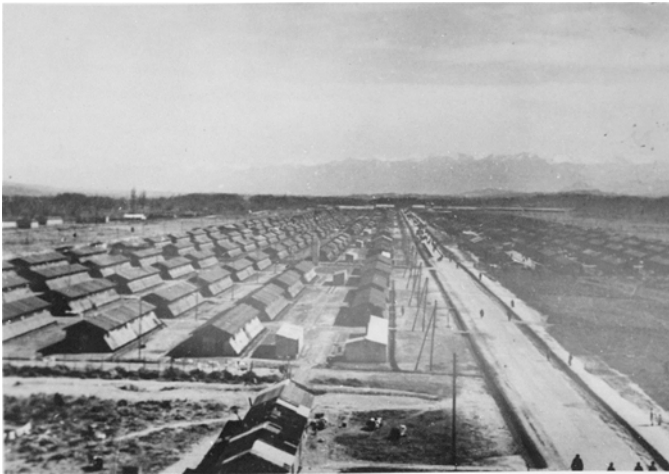
Figure 2: Photo of Gurs
