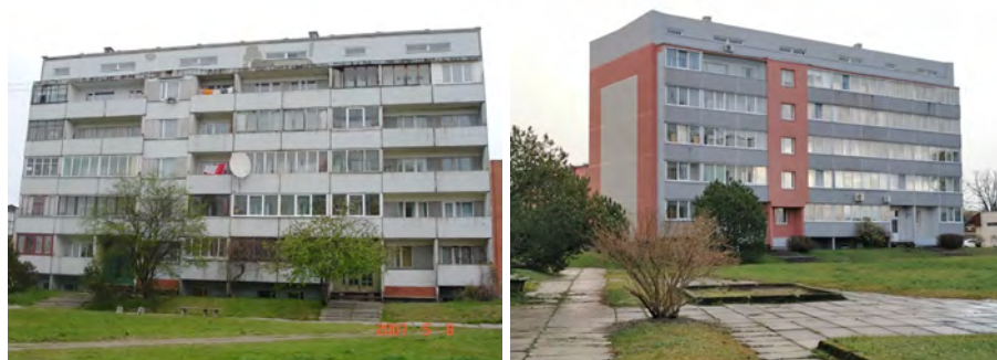
Figure 1 + 2: A typical Series 104 apartment building from the 1970s before and after refurbishment (more than 60% energy savings). The building in Jelgava was one of the first to undergo complex refurbishment and received the award in the “The Best Energy Efficient Building in Latvia” competition in 2010.
