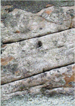
Lagerparallele Risse
