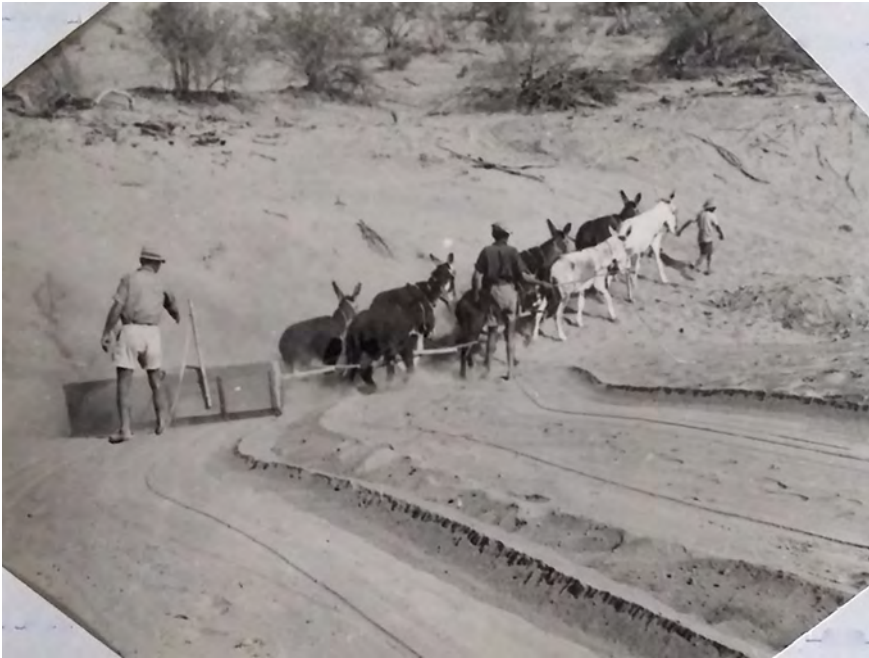
Fig. 4: Land levelling operations on Niemöller's farms, 1950s (Photo: GNPA, Pofadder).
