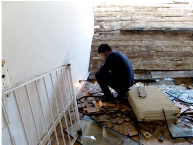
Figure 5.7: Cutting metal pipes 10
