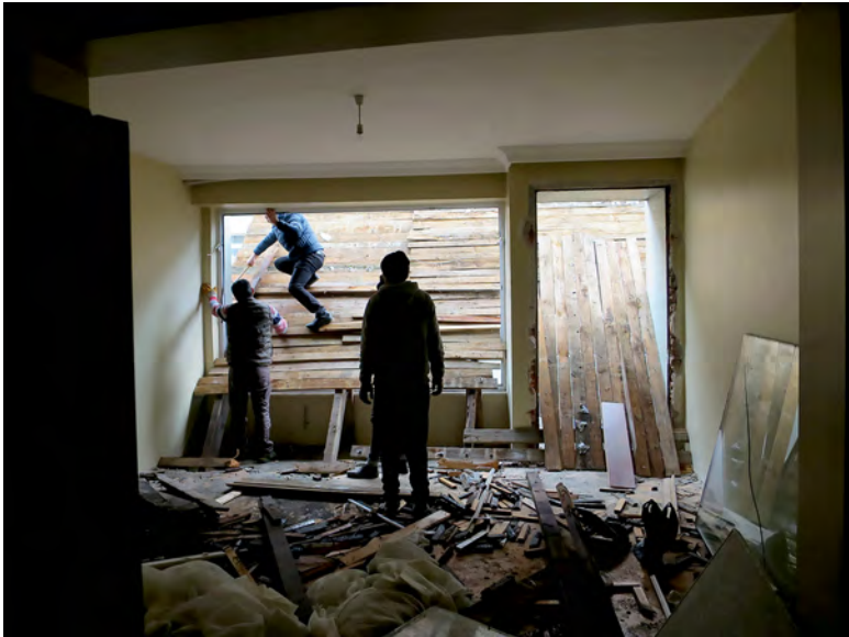
Figure 5.6: Installing the debris slide 9
