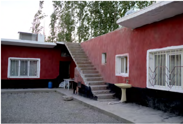
Figure 5.12: The house belongs to Engin's father. The washbasin was salvaged from a flat in Istanbul. On summer nights, they live on the terrace.
