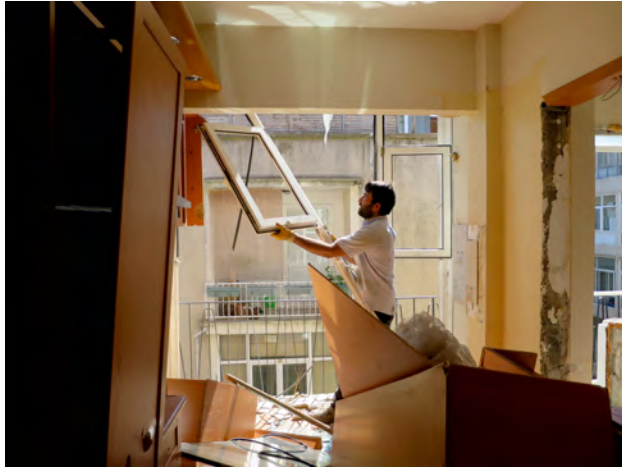
Figure 5.8: Dismantling PVC frames 11
