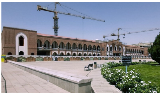
Figure 53: The ongoing reconstruction project of the Baladiyeh
