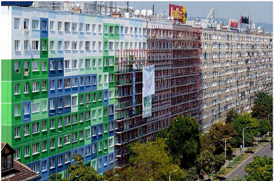
Figure 5: Installing the exterior insulation on the largest prefabricated building in Hungary, the so-called Village House in Óbuda, Budapest.
