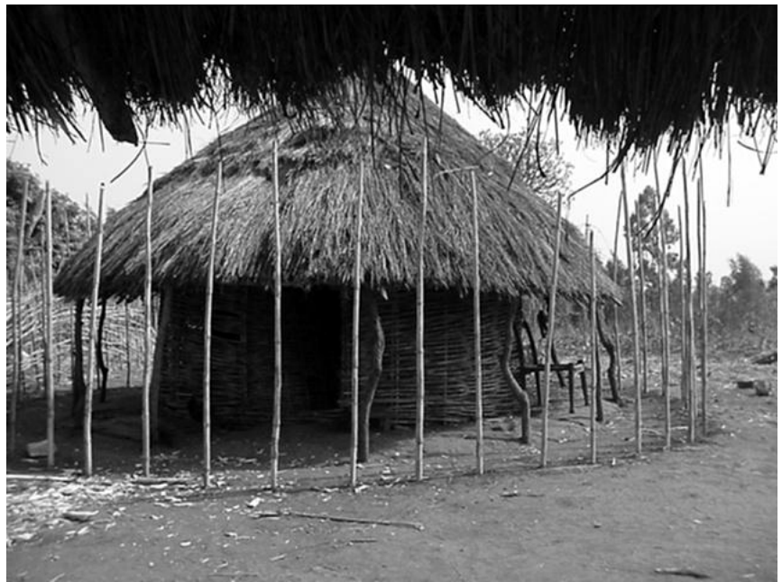
Fig. 7: Building an external ring to enlarge a kitchen and transforming it in a main house. Gundul (Asosa).
