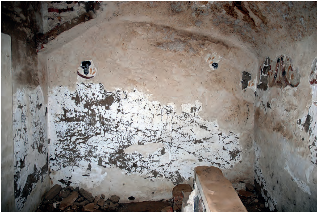
Abb. 13: Erdgeschoss, 2. Raum, Westwand; 2008
