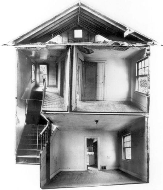
Abb. 22: Gordon Matta-Clark, Splitting, 1974
