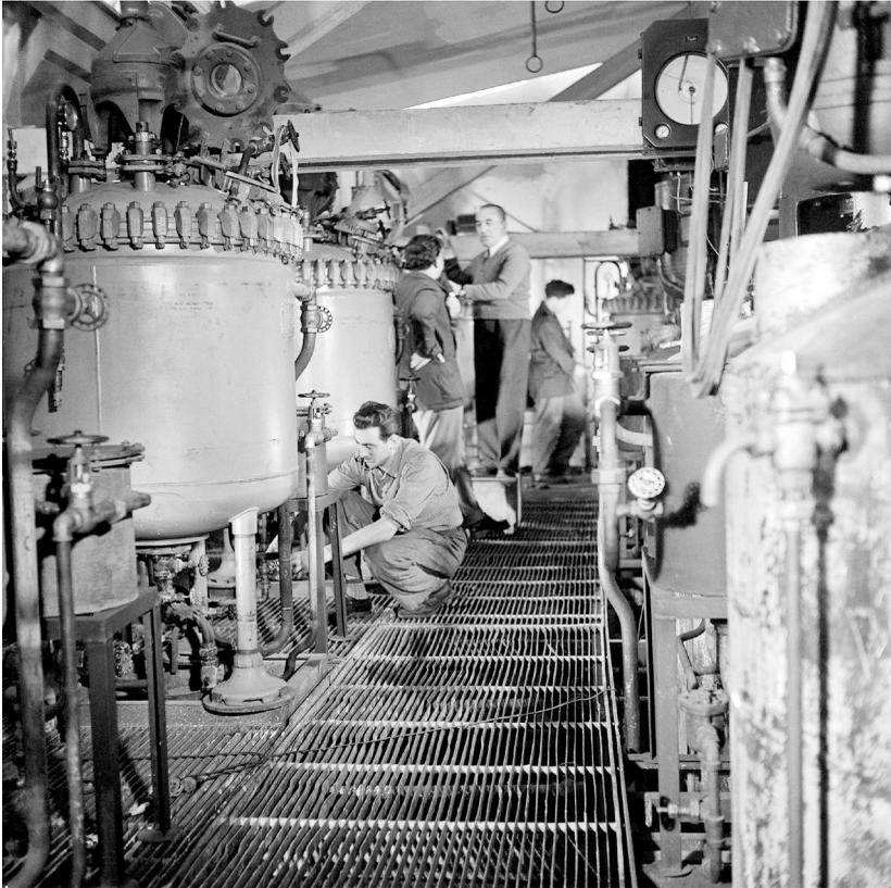
**Figure 1.** Upgrading the penicillin plant in Zemun in late 1953. The small tanks, in which a mixture is prepared for final fermentation in large tanks, were also part of the original Merck factory (Courtesy of the United Nations, UN Photo/GG, no. 156110.).
