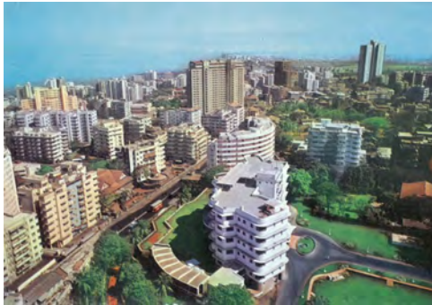
Fig. 38: North-western suburb of Mumbai, residential buildings built in the 1970s.
