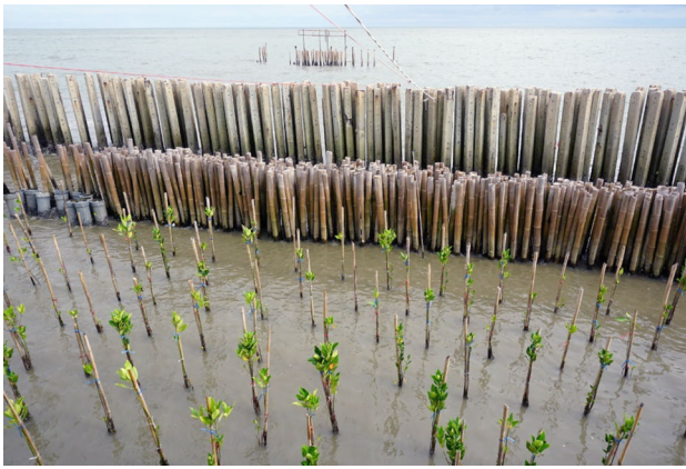
Figure 5: Coastal protection measures in Bang Khun Thian.
