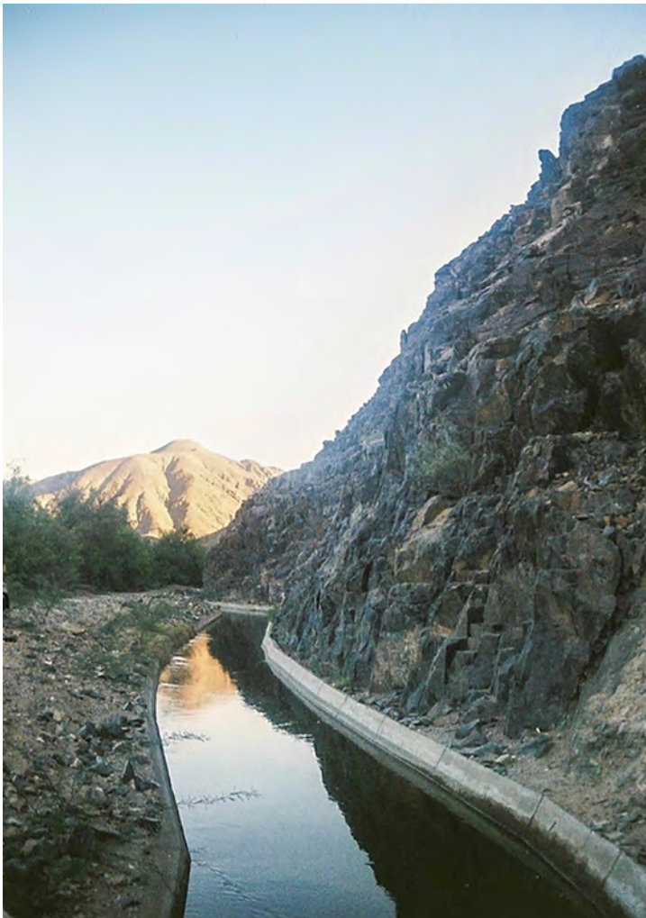
Fig. 2: Canal at proposed site of Noordoewer/Vioolsdrift dam (January 2020) 35mm film (Sindi-Leigh McBride private collection).
