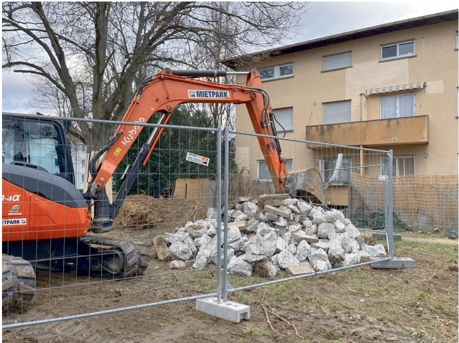
Picture 3: Construction work in the estate
