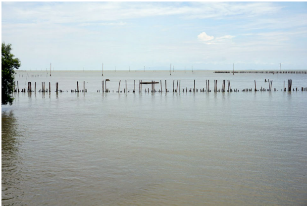
Figure 3: Submerged electricity pylons in Ban Khun Samut Chin.
