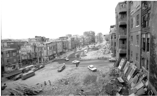
Figure 4.9: A general view of the demolition and salvage activity in Tarlabası. On the right, reclaimed doors are leaning on the buildings. On the left, there is a heap of wood
