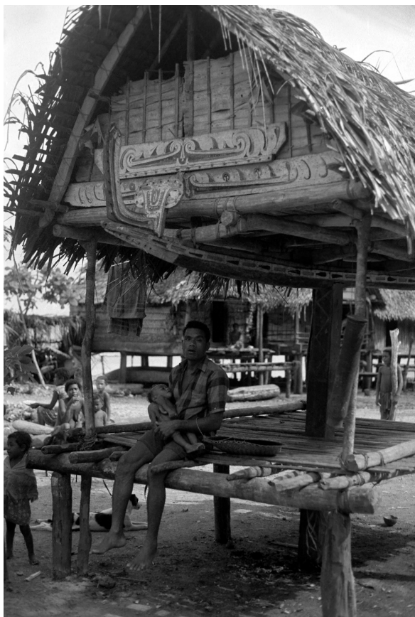
Fig. K8: Right front of the bomiyoyeva , decorated with two horizontal boards ( tataba ) mounted against the plaited front ( ninwa ).
