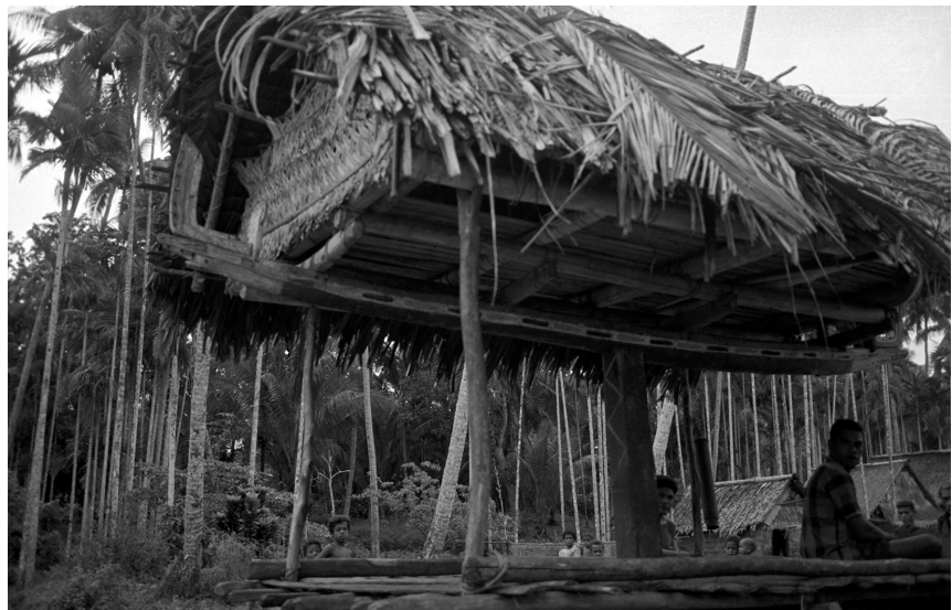
Fig. K4: Left rear side view, showing the decorated side of the horizontal beam ( waga ) and its rear canoe-prow with a carved tip ( pusa ), a transverse canoe-board ( lagim ) and a very unusual sagittal canoe-board ( tabuya ). At the left one of the two outriggers of the canoe supporting the upper floor ( bomakau ) of the loft ( tatom ).
