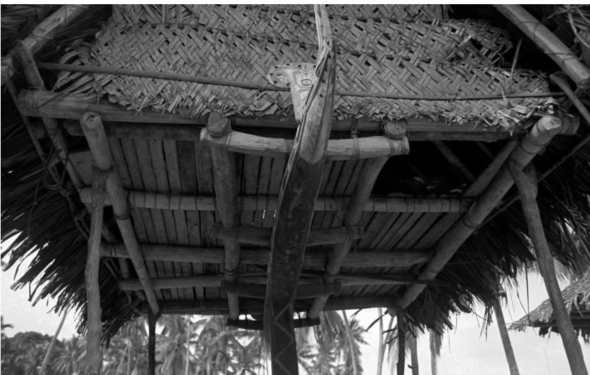
Fig. K5: Right rear side view. The horizontal beam ( waga ) is supported by the square central post ( kokola bwala ). The waga shows carved decorations ( tara-papa ) over its full length. The only access ( kaukweda ) to the loft ( tatom ) is just visible at the proximal corner of the building.
