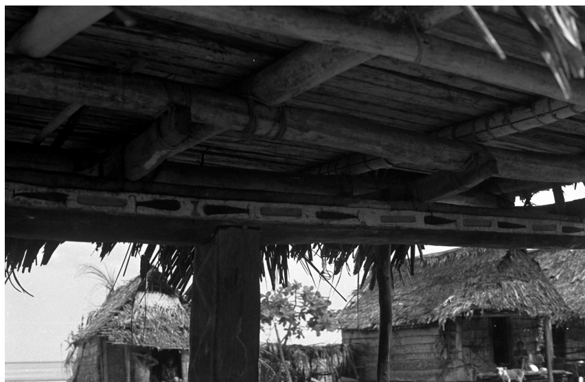
Fig. K7: Close-up of the joint where the vertical post ( kokola bwala ) carries the horizontal central canoe-shaped beam ( waga ). Note that both the post and the hole in the waga are square, preventing any rotation of the roof ( katua ) of this bomiyoyeva , of its floor ( bomakau ) or canoe-shaped beam.
