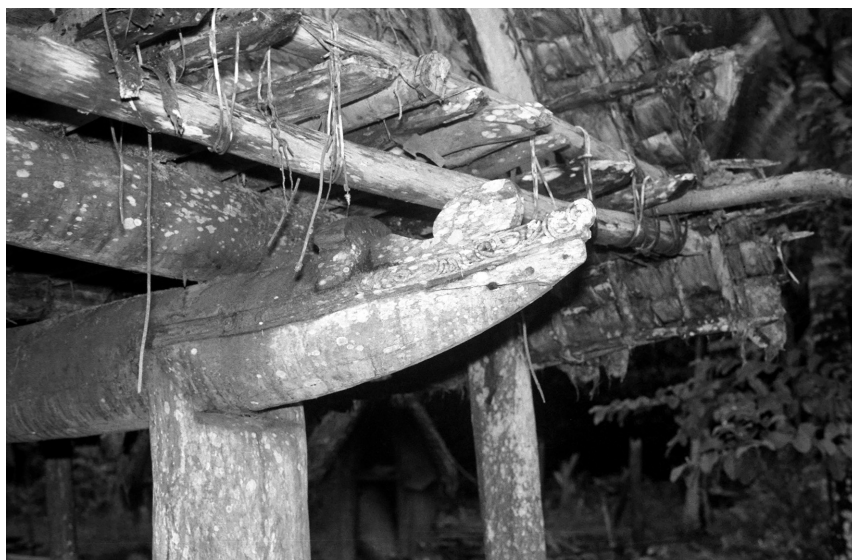
Fig. L4: As L3. Note the carved decoration on the side of the canoe ( keta'ula ). Three large horizontal beams ( pou ) which rest on the keta'ula support the floor ( ke-bila ) of the loft ( tatom ).
