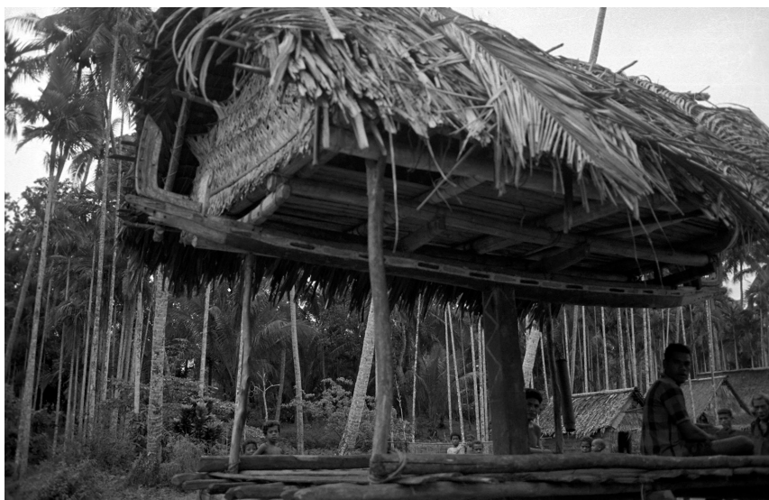
Fig. K14: Right rear view of the rear end of the canoe-shaped beam ( waga ) and its canoe-prow.
