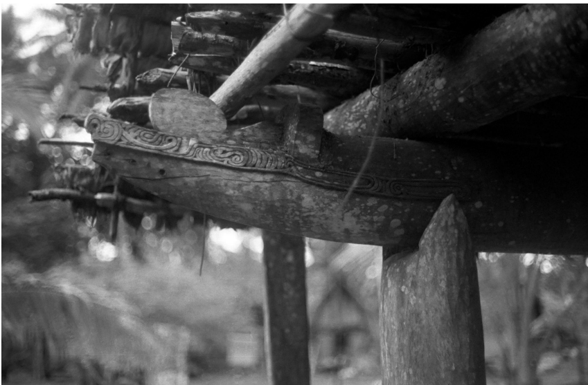
Fig. L3: Details of the front end of the horizontal canoe-shaped beam ( keta'ula ) resting on the frontal post ( kokola ) which features a carved canoe-tip ( pusa ) and a small (undecorated) sagittal canoe-board ( tabuya ), but no transverse board ( lagim ).
