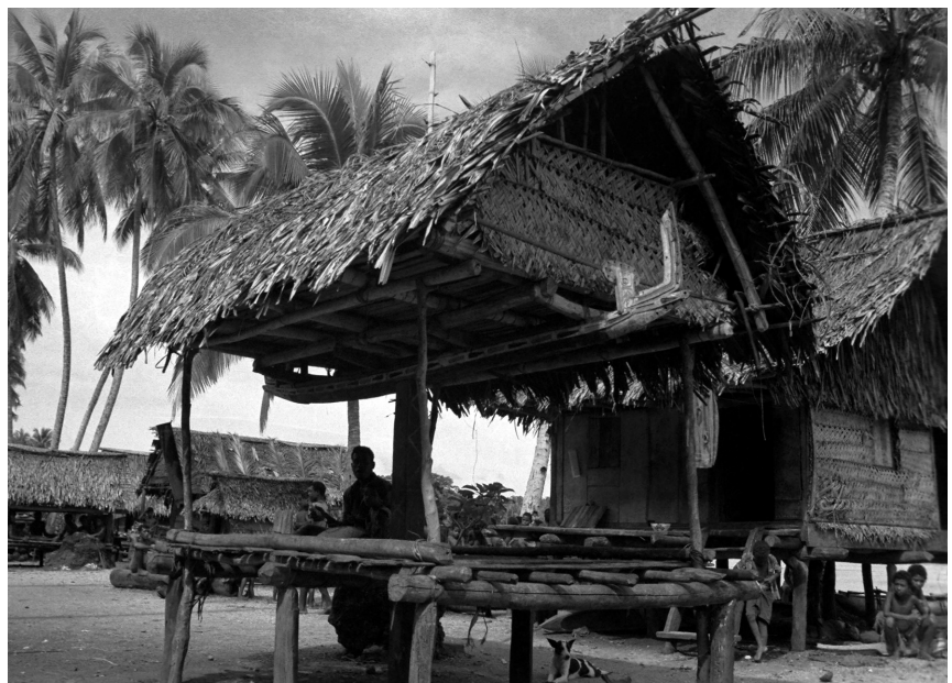
Fig. K13: Left rear view of the bomiyoyeva , showing the left rear end of the canoe-shaped beam ( waga ) with its rear canoe-prow consisting of the canoe-tip ( pusa ), a transverse board ( lagim ) and an – again unusually high – sagittal board ( tabuya ).
