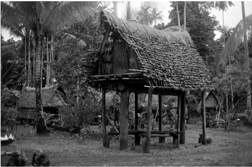
Fig. L2: As L1, rear view. There are 2 large central posts ( kokola ) supporting the canoe-shaped horizontal beam ( keta'ula ). The building features a lower platform ( kabodaga ) as well as an upper platform ( kebila ) which is the floor of the loft ( tatom ). To the left and right of the keta'ula six vertical posts ( kainubiluma ) – which are much smaller than the kokola – stabilize the ends of 3 horizontal beams ( pou ) which rest on the keta'ula and which support the floor of the loft ( tatom ).
