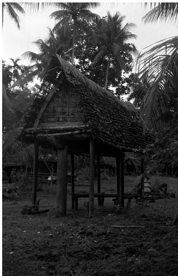
Fig. L1: Frontal view of Chief Tolosi's dilapidated bomduvadova in the center ( baku ) of Labai village. Note the remnants of the lower platform ( kobudaga ) (Labai, Kiriwina Island, 1971).
