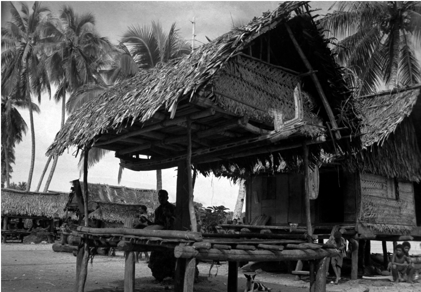
Fig. K4: Left rear side view, showing the decorated side of the horizontal beam ( waga ) and its rear canoe-prow with a carved tip ( pusa ), a transverse canoe-board ( lagim ) and a very unusual sagittal canoe-board ( tabuya ). At the left one of the two outriggers of the canoe supporting the upper floor ( bomakau ) of the loft ( tatom ).
