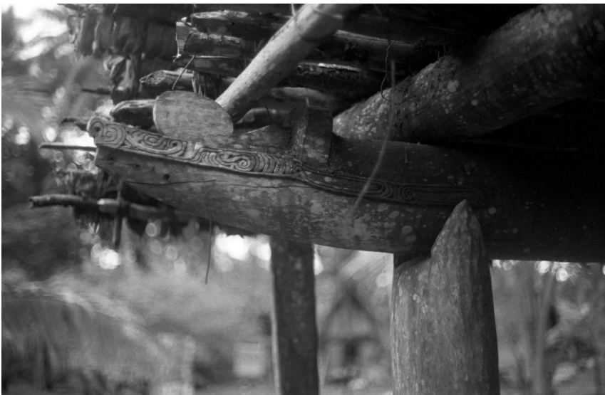
Fig. L3: Details of the front end of the horizontal canoe-shaped beam ( keta'ula ) resting on the frontal post ( kokola ) which features a carved canoe-tip ( pusa ) and a small (undecorated) sagittal canoe-board ( tabuya ), but no transverse board ( lagim ).
