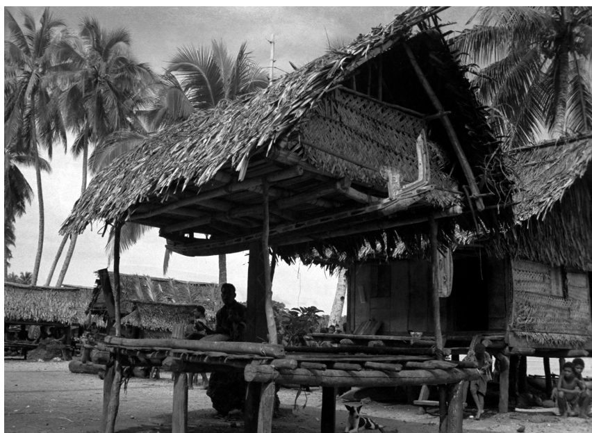
Fig. K13: Left rear view of the bomiyoyeva , showing the left rear end of the canoe-shaped beam ( waga ) with its rear canoe-prow consisting of the canoe-tip ( pusa ), a transverse board ( lagim ) and an – again unusually high – sagittal board ( tabuya ).
