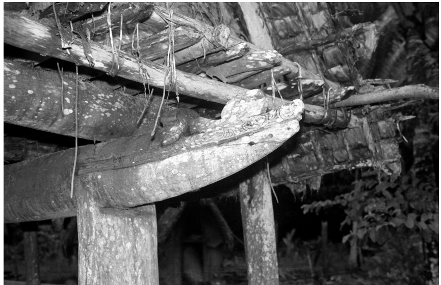
Fig. L4: As L3. Note the carved decoration on the side of the canoe ( keta'ula ). Three large horizontal beams ( pou ) which rest on the keta'ula support the floor ( ke-bila ) of the loft ( tatom ).
