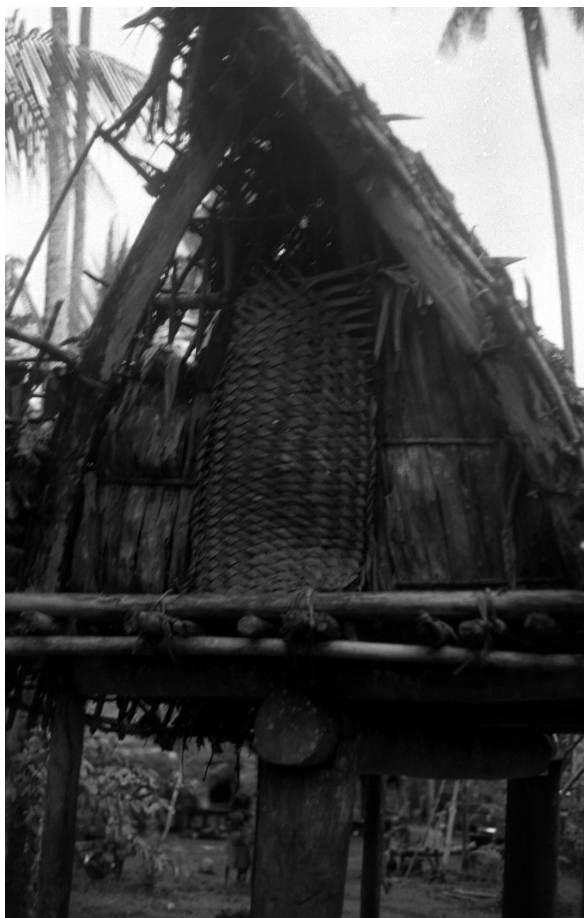
Fig. L5: Rear view of Chief Tolosi's bomduvadova . The rear end of the central horizontal beam ( keta'ula ) is not carved. The only entrance to the loft ( tatom ) is closed off with a woven mat ( yoyu = taluguma ). The roof ( katua ) is badly damaged.
