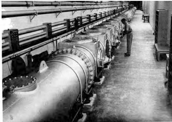
Pressurized spark range is a steel tube, 3 feet in diameter, 313 feet long. A 20-mm. gun at one end fires models into sand butt at other. Spark stations in between photograph the flight.
