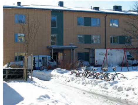
Figure 6-9: Moving back of temporarily evacuated residents in a revitalization project to the refurbished building. Source: Alingsåshem
