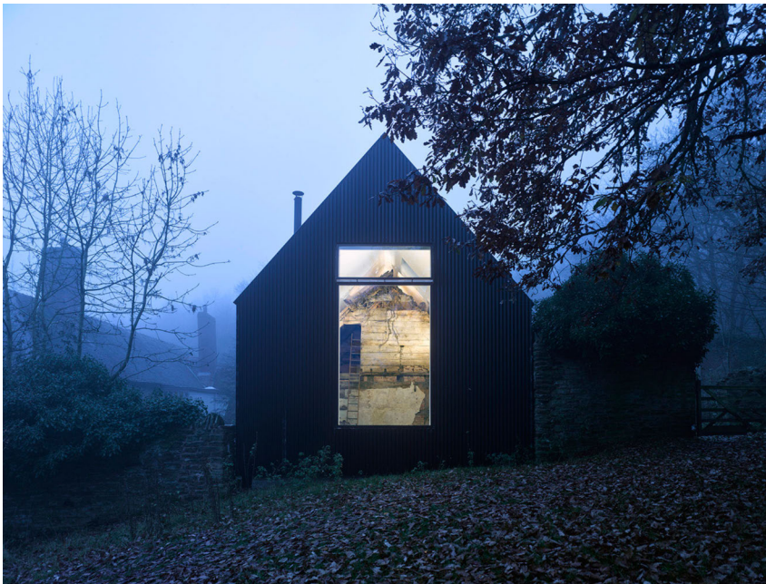
Figure 10: Croft Lodge, exterior of completed project, Leominster UK. (Kate Darby and David Connor; image courtesy of James Morris).
