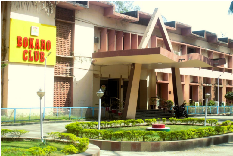
Figure 5: Bokaro Club, Bokaro Steel City, March 2023.
