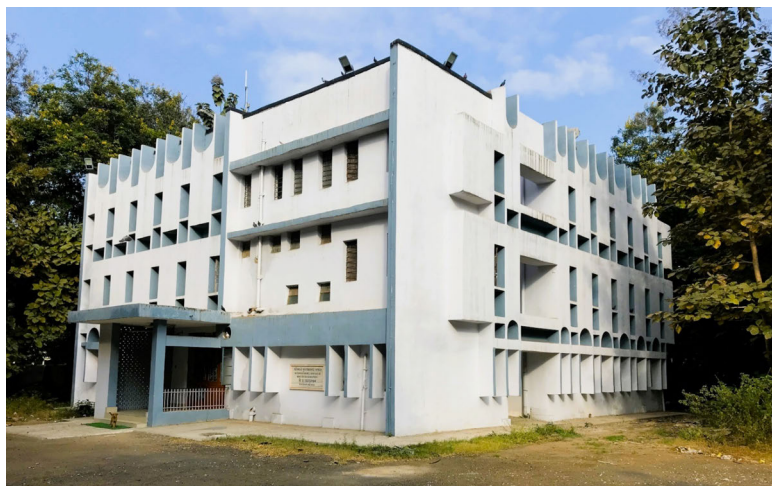
Figure 4: Central Library, Bokaro Steel City, November 2023.
