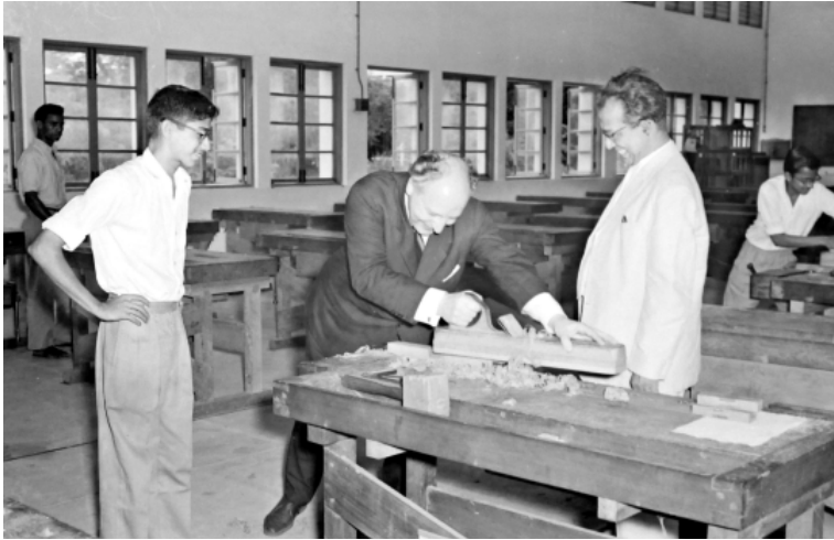
Fig. 1: Minister of Economic Cooperation and Development of the Federal Republic of Germany, Walter Scheel (center), visibly enjoying woodwork in the carpentry workshop during his visit to IIT Madras on 4 December 1963. The man in the white suit on the right is Professor Bibhutibhushan Sengupto, the first director of IIT Madras. Photographed by Cadambi Gourishankar (Photo: Heritage Centre, IIT Madras).
