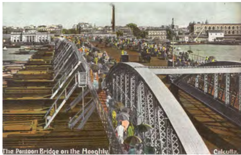
Fig. 14: Kolkata, The old pontoon bridge (1874).
