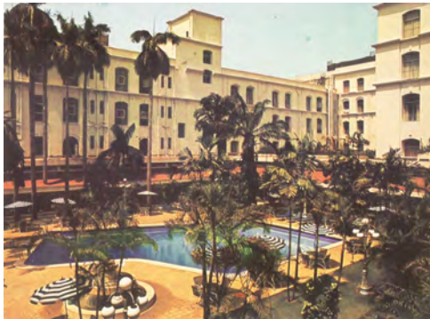
Fig. 40: New Delhi, Interior courtyard of the Oberoi Hotel in the 1970s.
