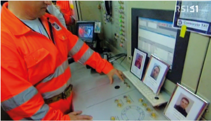
Fig. 36: The tunnel boring machine called Sissi, on the south side of the tunnel tube, is tackling the last wall. On the control panel photographs of the people who died in working accidents are visible.
