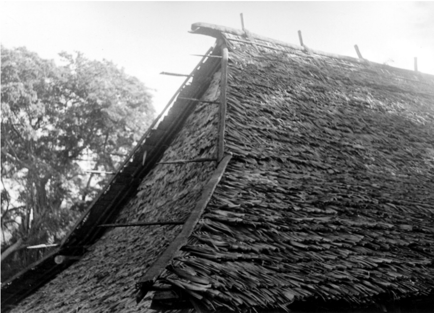
Fig. 3: Wooden spears in the roof of the Lewotala Temple.
