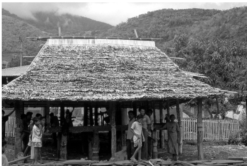
Fig. 5: Riang Kĕmie Temple under construction 1995.
