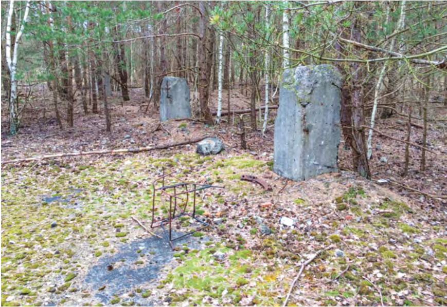
Fig. 4: Concrete floor at Fertigungshalle 1 (F1) (6 September 2021). Photo by P. Schneider and C. Röhl.
