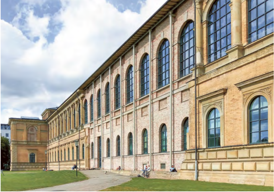
Fig. 3: Alte Pinakothek Munich – Hans Döllgast’s intervention on the south façade consisting of a structure of steel columns supporting the roof and the subsequent closure of the gap with re-used bricks, photo 2021.
