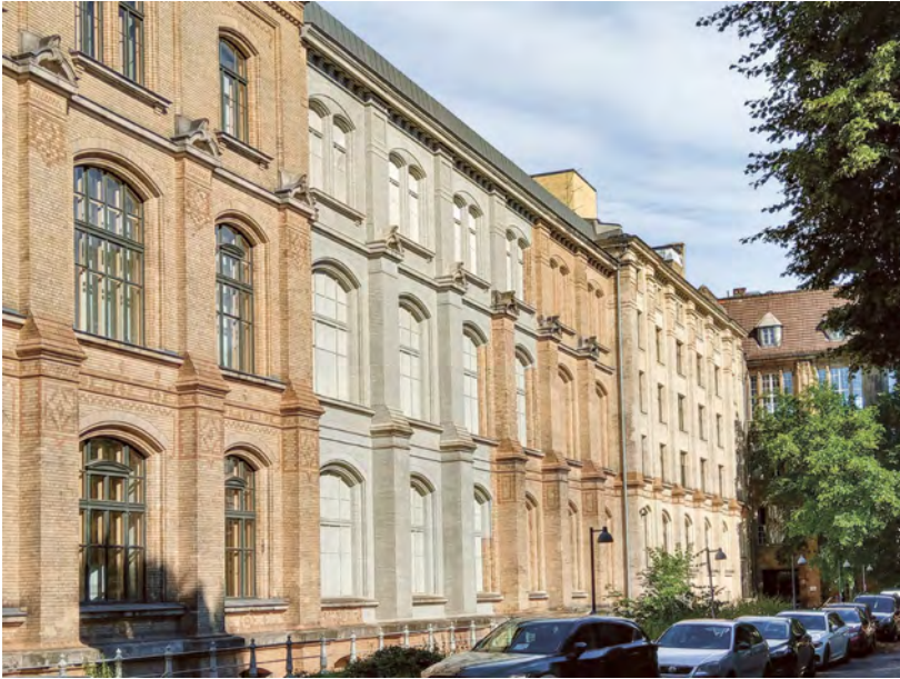
Fig. 7: Natural History Museum Berlin – restored east wing, Diener & Diener Architekten, photo 2021.
