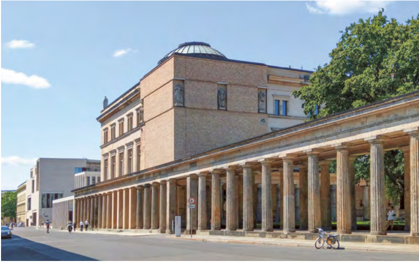
Fig. 6: Neues Museum Berlin – south-east façade with newly built corner risalto and rebuilt south colonnade, David Chipperfield Architects, photo 2021.
