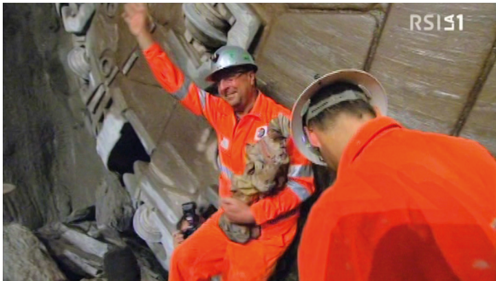
Fig. 39: St. Barbara and Hubert Bär after having crossed the new passage through the Gotthard.
