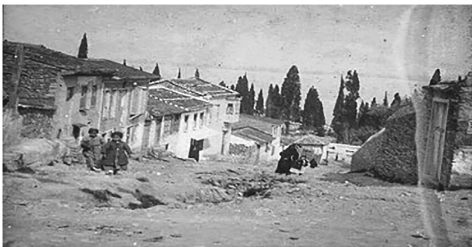
Figure 2: General view of Apano Mahala (Upper Neighbourhood) of Smyrna – a poor neighbourhood (source: Levantine Heritage Foundation)
