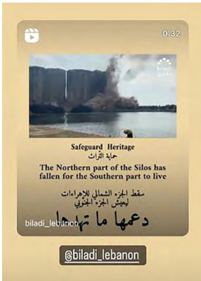
Fig. 5.24: Biladi NGO (@biladi_lebanon), ‘The Northern Part of the Silos Has Fallen for the Southern Part to Live’, Instagram, 31 July 2022.
