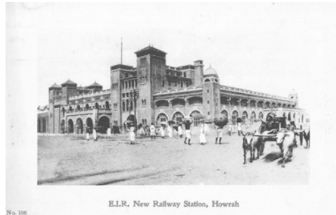
Fig. 33: Howrah, New Railway Station.
