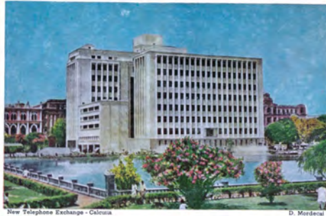
Fig. 34: Kolkata, New Telephone Exchange.
