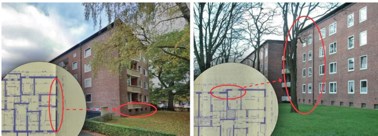
Figure 2: Example of Diederhofer Straße; discrepancies between planning documents and actual building.
