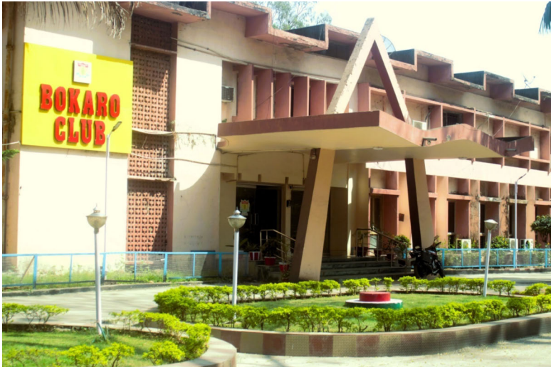
Figure 5: Bokaro Club, Bokaro Steel City, March 2023.
