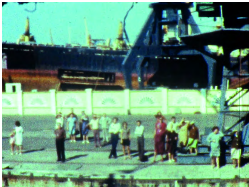
Figure 19: Mariupol Port, viewed from a ship
