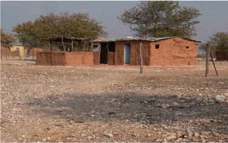
Figure 5: House built with local materials
