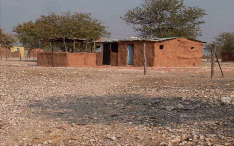
Figure 5: House built with local materials
