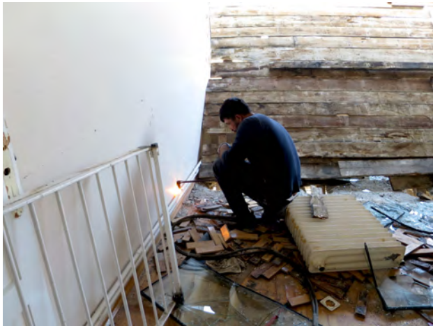
Figure 5.7: Cutting metal pipes 10
