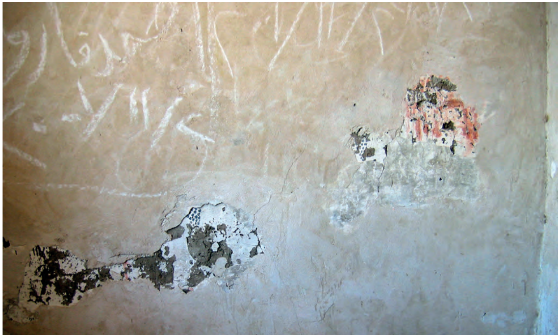
Abb. 10: Erdgeschoss, 1. Raum, Detail Westwand; 2005
