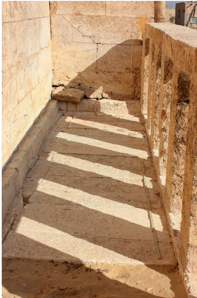
Fig. 5: Preserved pavement between naos and balustrade; 2015
