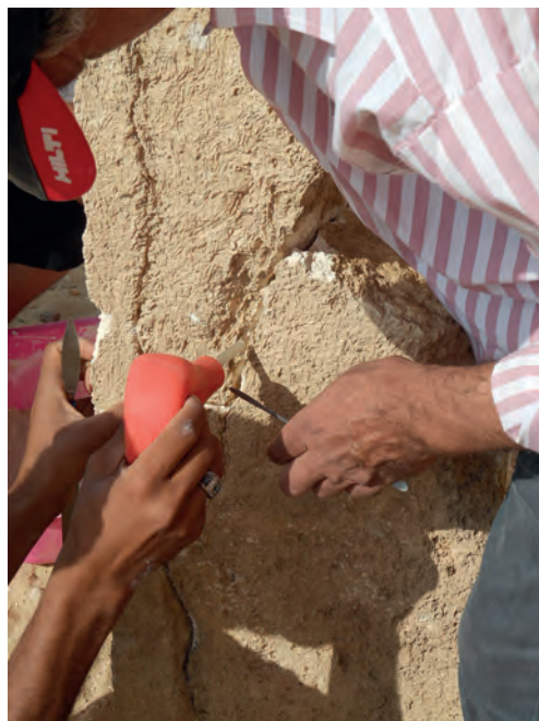
Fig. 13: Closing gaps with the help of lime mortar; 2015
