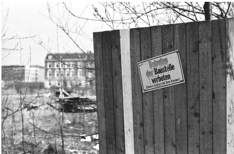
Fig. 4: Asmus Henkel, Building site, 1982 © Asmus Henkel
