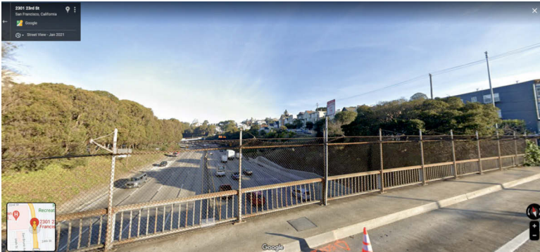
Figure 1: The 23rd Street overpass above Highway 101 in San Francisco as captured by Google Street View in January 2021.
