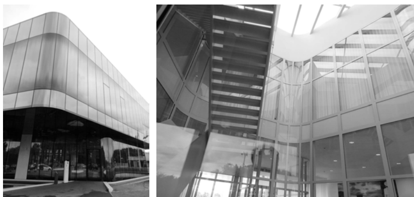
Figure 11: Entrance to the Maasbracht control room. Figure 12: Courtyard of the Maasbracht control room, with the curtains of the control room on the first floor closed.
