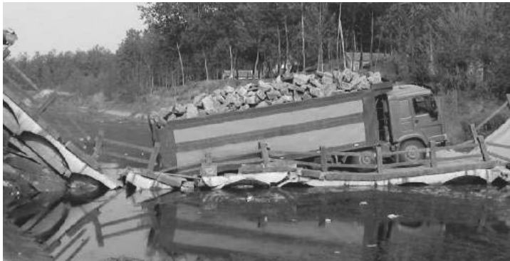
Fig.3 : China Jiangsu net- Overloading truck damaged the bridge
