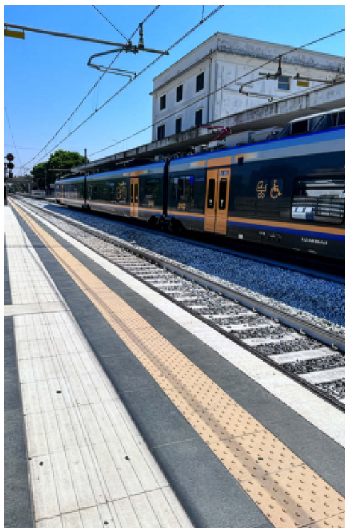
Fig. 50: Train station of Ostuni. The photo shows the guiding system (guiding lines and stop signals).
