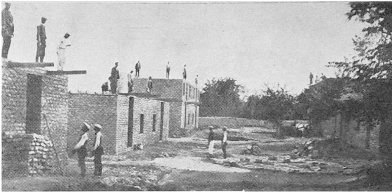
Figure 5.8. Settlement in Perçenç (Akçakiraz), built in 1935. 83
