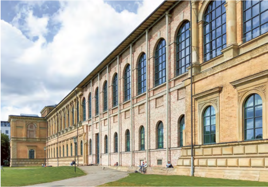
Fig. 3: Alte Pinakothek Munich – Hans Döllgast’s intervention on the south façade consisting of a structure of steel columns supporting the roof and the subsequent closure of the gap with re-used bricks, photo 2021.
