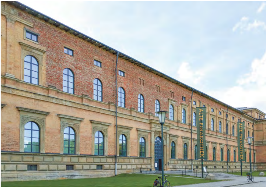
Fig. 4: Alte Pinakothek Munich – Hans Döllgast’s reintegrated north façade with bare re-used bricks and lack of decorative elements, photo 2021.
